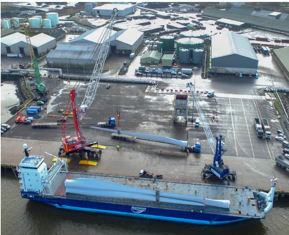
Figure 89. Shannon Foynes, Phase 1 of the Jetty expansion programme at Foynes. Photo courtesy of the Department of Transport, Tourism and Sport
