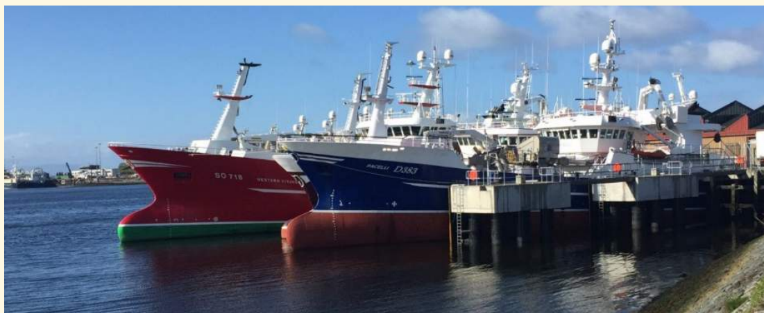
Figure 80. Vessels berthed alongside the completed Mooring Dolphins funded as part of the Killybegs Landing Pier Fendering Project under the Fishery Harbour Centre and Coastal Infrastructure Development Programme. Photo courtesy of DAFM
